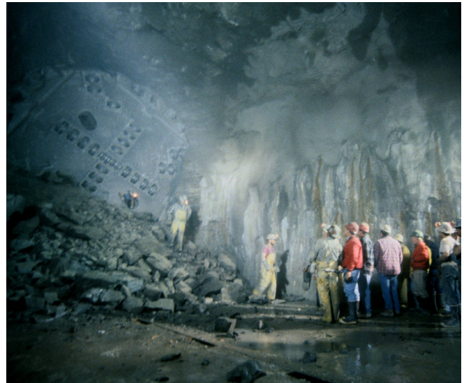
Work got underway in the 1970s to bore through limestone about 300 feet below ground to form the tunnels that would allow the MWRD to store and convey water throughout the Chicago area's 375-square miles of combined sewer systems.
