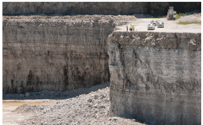
From below ground in the tunnels to high above the rim of the reservoirs, the MWRD has documented the different phases of the Tunnel and Reservoir Plan (TARP). The MWRD bored through more than 100 miles of tunnels, then lined them with concrete, installing drop shafts, gates and pumping stations and other structures, and then began the next phase of excavating reservoirs, including the Thornton Composite Reservoir (middle row, bottom right) and McCook Reservoir (bottom left).
