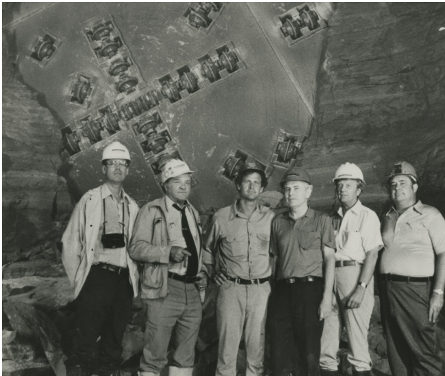
Work got underway in the 1970s to bore through limestone about 300 feet below ground to form the tunnels that would allow the MWRD to store and convey water throughout the Chicago area's 375-square miles of combined sewer systems.
