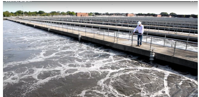
MWRD Commissioner Marcelino Garcia stands before aeration tanks at the Stickney Water Reclamation Plant.
