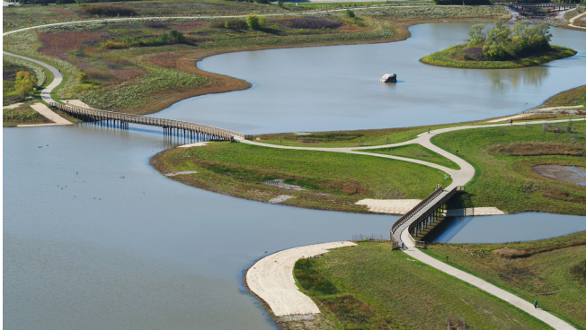
As part of the Buffalo Creek Reservoir Expansion project, seven new timber boardwalks were installed and pedestrian paths were relocated and reconstructed to remove them from inundation during the 10-year storm event.
