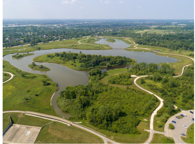
The Buffalo Creek Reservoir Expansion Project increased storage capacity to alleviate flooding for downstream communities, while at the same time improving public recreation amenities at Buffalo Creek Forest Preserve. The MWRD increased the existing reservoir volume by approximately 180 acre-feet to account for an additional 58.6 million gallons of flood storage.
