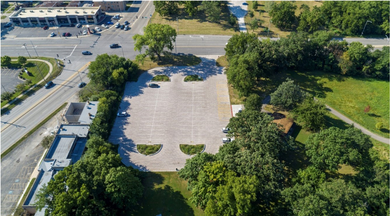
A new permeable parking lot at Schuth's Grove in the Forest Preserves of Cook County was funded by the MWRD to mitigate flooding, protect local water quality and make an attractive space that increases accessibility to the Des Plaines River.
