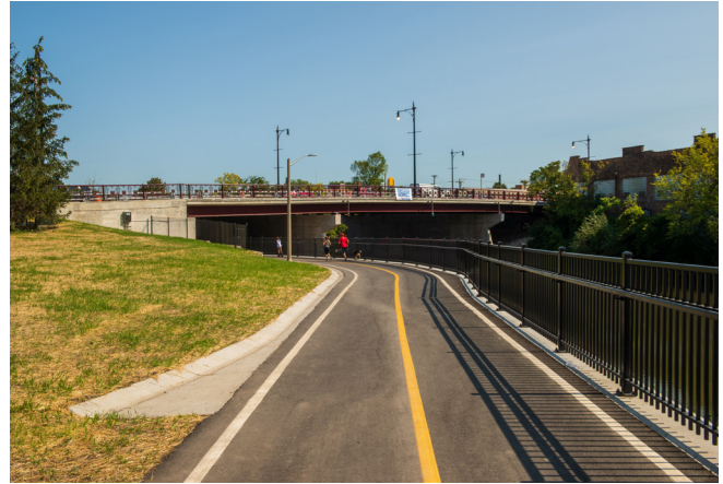
The new Irving Park Road Bridge and 312 RiverRun trail
