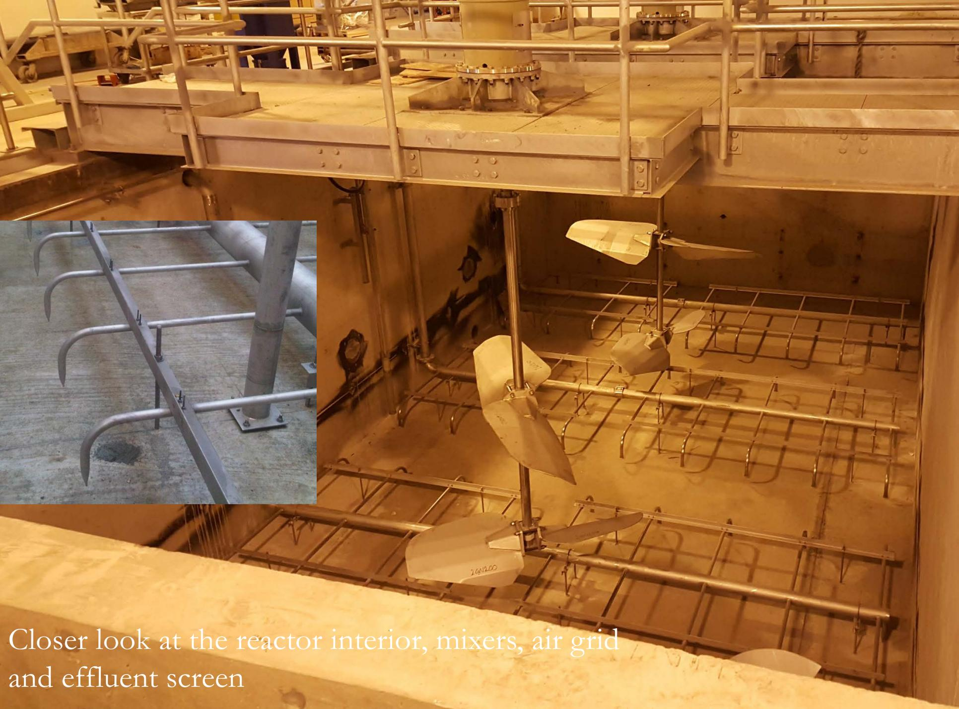
Closer look at the reactor interior, mixers, air grid and effluent screen
