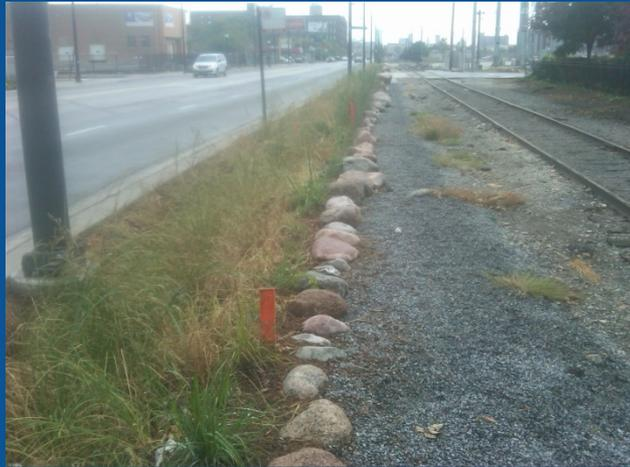
In 3 years of monitoring, the bioswale never returned water to the catch basin through the underdrain.
