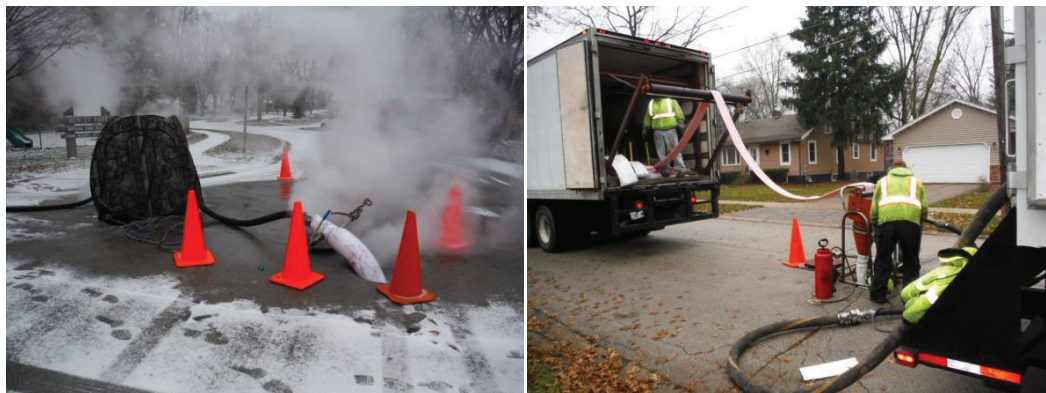
Figure 8.19: Cured-in-Place Pipe (CIPP) Lining
