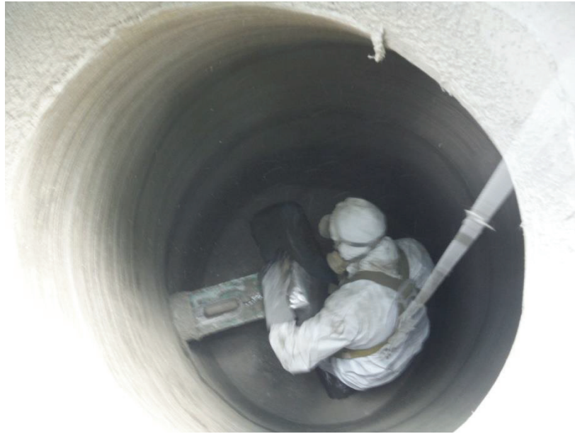
Figure 8.18: Manhole Rehabilitation by Cementitious Lining
