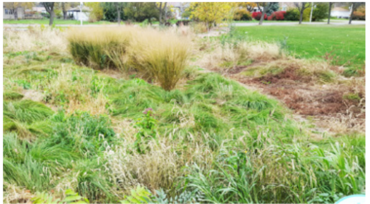
A bioswale created through a partnership with MWRD stormwater engineering to alleviate flooding in this park.
