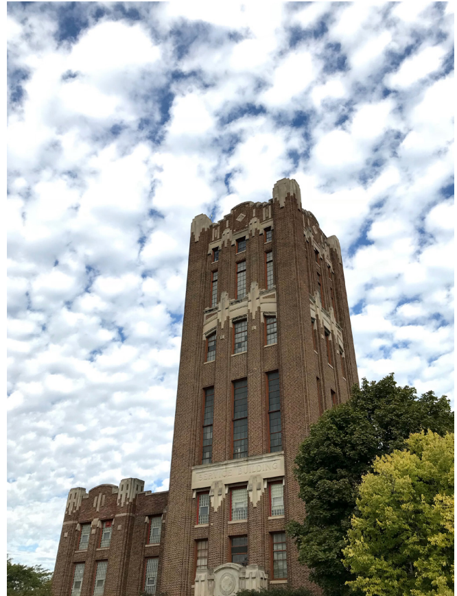
The O'Brien Service Building was one of the featured buildings on the architecture tour. It was constructed in 1928 and houses the boilers for plant heating, the storeroom, and all trades shops. Inside the tall tower is a large water tank that has a 150,000 gallon capacity.
