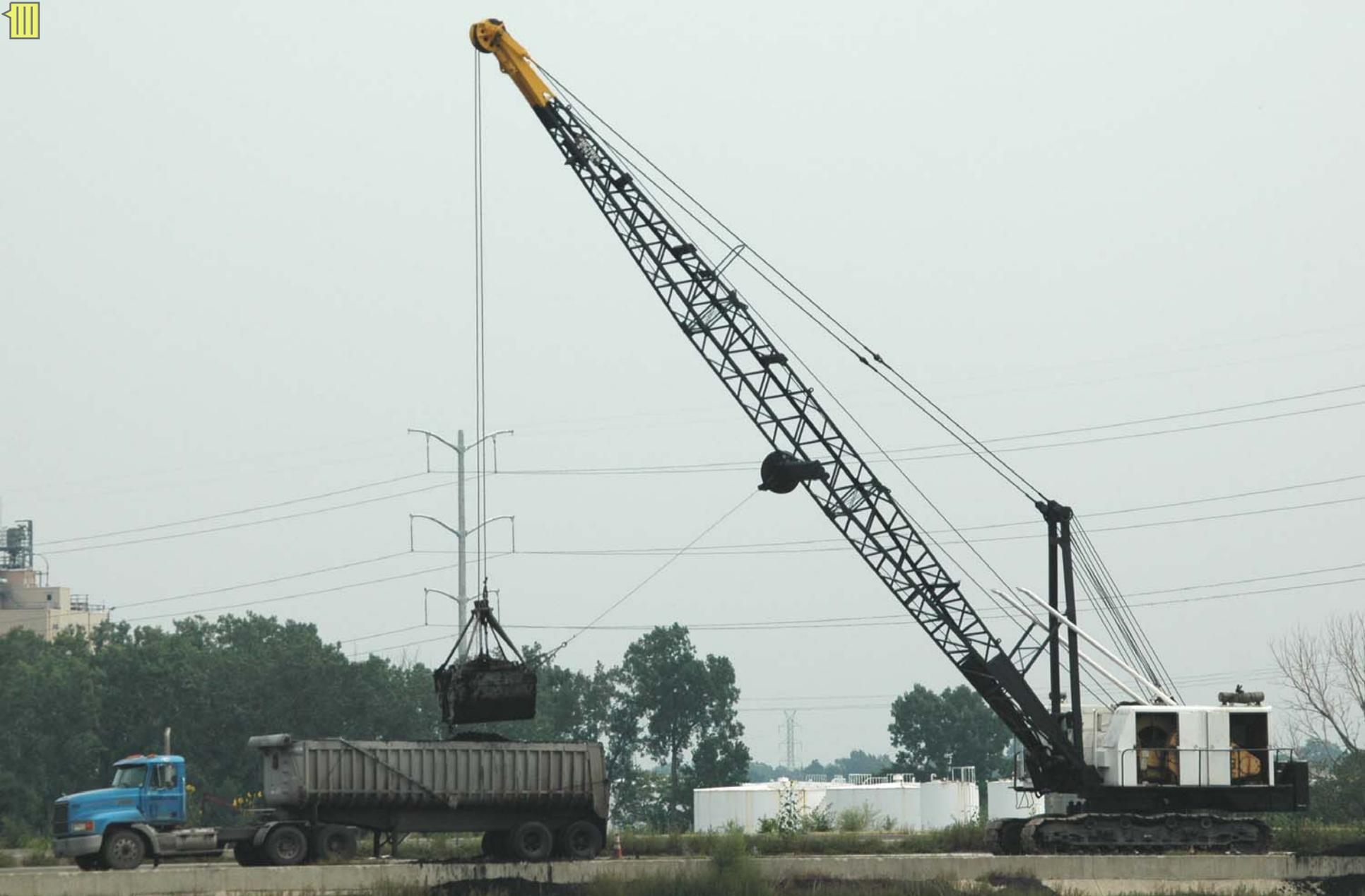
**Crane with Clamshell Bucket Outloading a Lagoon for Transportation to Drying Site**
