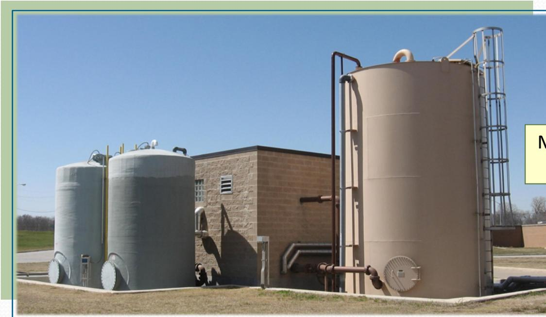
Mix tank on right, two batch tanks on left
