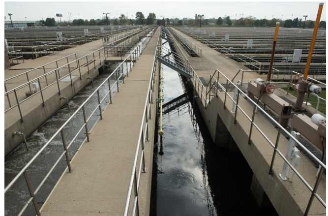
The MWRD's Kirie Water Reclamation Plant in Des Plaines is commemorating 40 years of essential service to treat more than 50 million gallons of wastewater every day for more than 260,000 residents living in the northwest suburbs.
