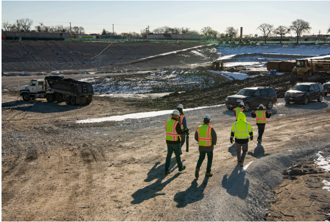
Workers survey Addison Creek Reservoir.
