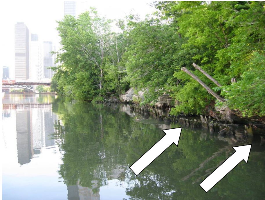
Figure 2-11: Bank Pocket Areas (indicated by white arrows) Created by a Decaying Wooden Seawall on the South Branch Chicago River (photo taken downstream of AWQM 39, 2008).
