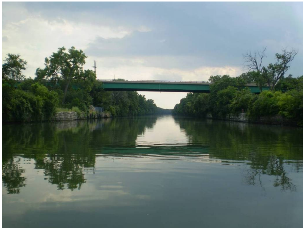
Figure 2-15: Most of the CAWS Waterways Were Constructed Without Floodplains, Like This Middle Portion of the Chicago Sanitary and Ship Canal (photo taken downstream of AWQM 41, 2008).
