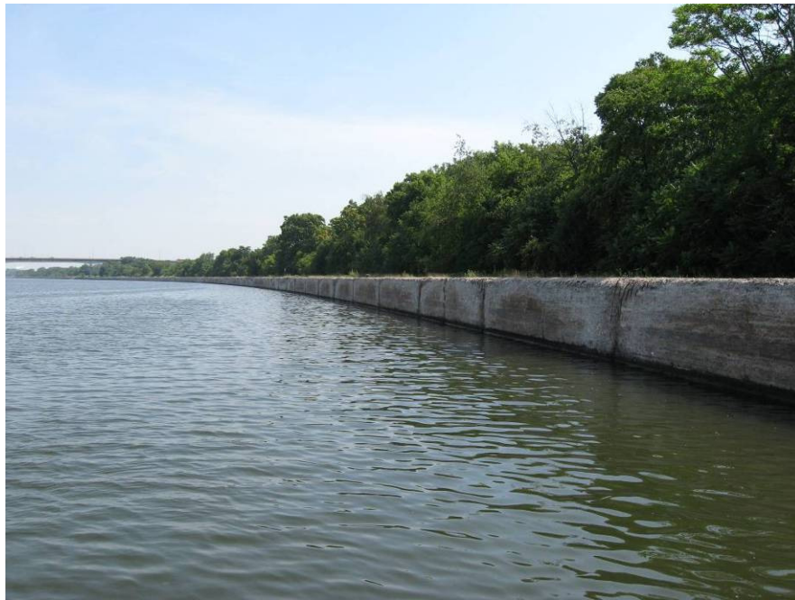
Figure 2-18: Many of the CAWS Reaches Completely Lack Littoral Zones by Design, Such as Seen Here in the Chicago Sanitary and Ship Canal (photo taken downstream of AWQM 48, 2008).
