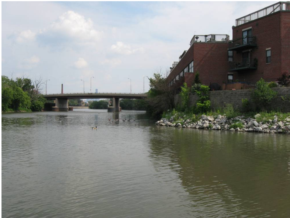
Figure 2-6: Riprap Banks in the North Branch Chicago River (photo taken near AWQM 73, 2008).
