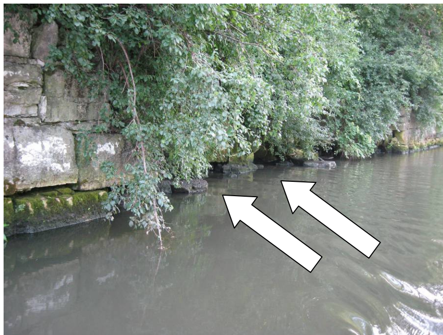
Figure 2-12: Bank Pocket Areas (indicated by white arrows) Created by a Gaps in Limestone Walls on the Chicago Sanitary and Ship Canal (photo taken downstream of AWQM 41, 2008).
