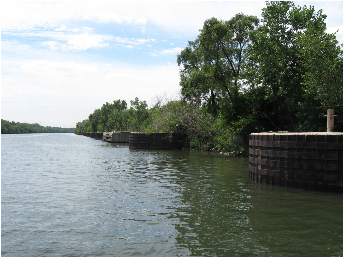
Figure 3-6: Examples of Manmade Structures (Dolphins) on the Chicago Sanitary and Ship Canal Near AWQM 41.
