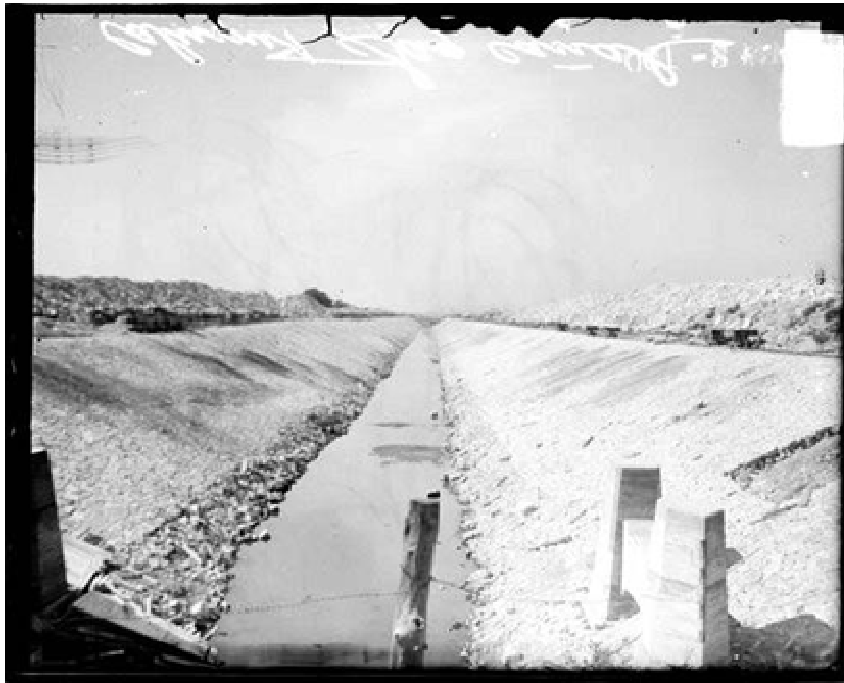
Figure 1-13: The Cal-Sag Channel under Construction, 1914 (Chicago Historical Society, The Electronic Encyclopedia of Chicago, 2005).
