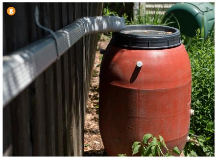
may need to tip the barrel some to allow more water out of the spigot before moving it.
