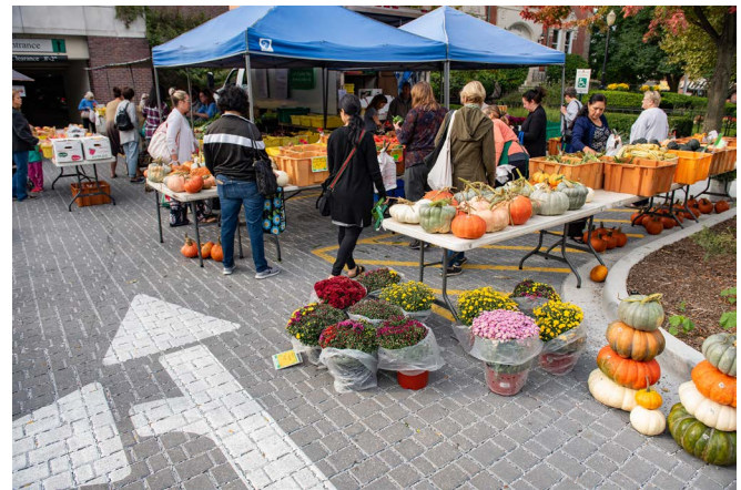
A farmer's market in La Grange, IL stands on a sustainable surface thanks to support from the MWRD. In 2019, the MWRD partnered with La Grange to install interlocking concrete permeable pavers that retain nearly 95,000 gallons of stormwater per rain event on two separate parking lots.
