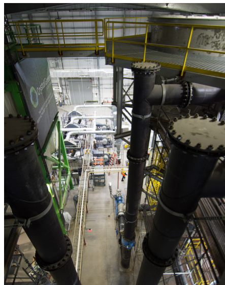
The MWRD's nutrient recovery facility with its three mega-sized reactors can recover more than 85 percent of the phosphorus and up to 15 percent of the nitrogen from the water cleaned by the plant.
