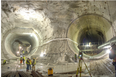
Construction at the confluence of the McCook Reservoir Connecting Tunnel (left) and Mainstream Tunnel (right)
