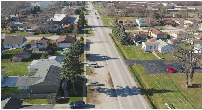
Homes along 135th Street east of Central Avenue in Crestwood will benefit from the installation of new storm sewers and other infrastructure investments made by the MWRD.
