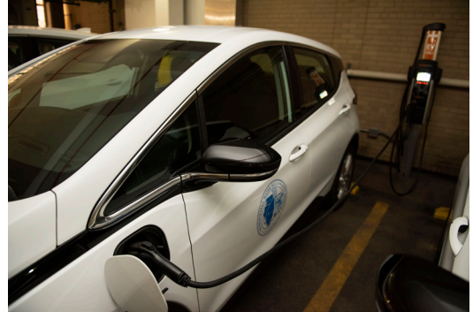
With the investment in seven new Chevy Bolts, the MWRD embarks on a new pilot study to test the performance of electric vehicles and charging stations for staff use.
