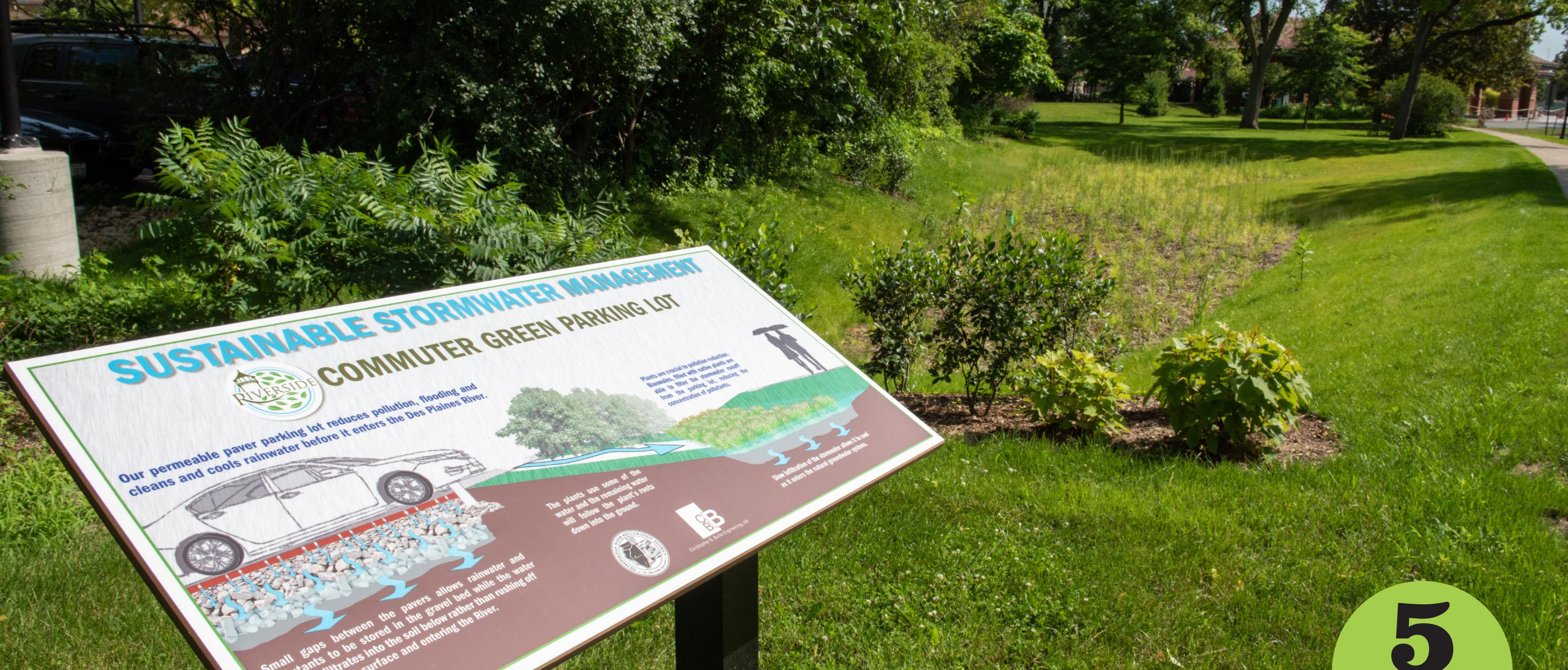
The District partnered with the Village of Riverside in 2019 to construct a new commuter parking lot and bioretention area that will provide parking for Metra commuters and more than 237,000 gallons of stormwater storage per rain event. The permeable parking lot and rain garden will reduce the current load to the combined sewer system and help alleviate flooding within the project area.
