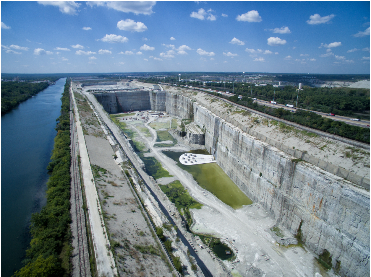
A nearly complete Stage 1 of the McCook Reservoir, one of three reservoirs in the MWRD's TARP system, is seen in this aerial photo from August 2017. Completed at the end of 2017, McCook Reservoir Stage 1 has the capacity to contain 3.5 billion gallons.
