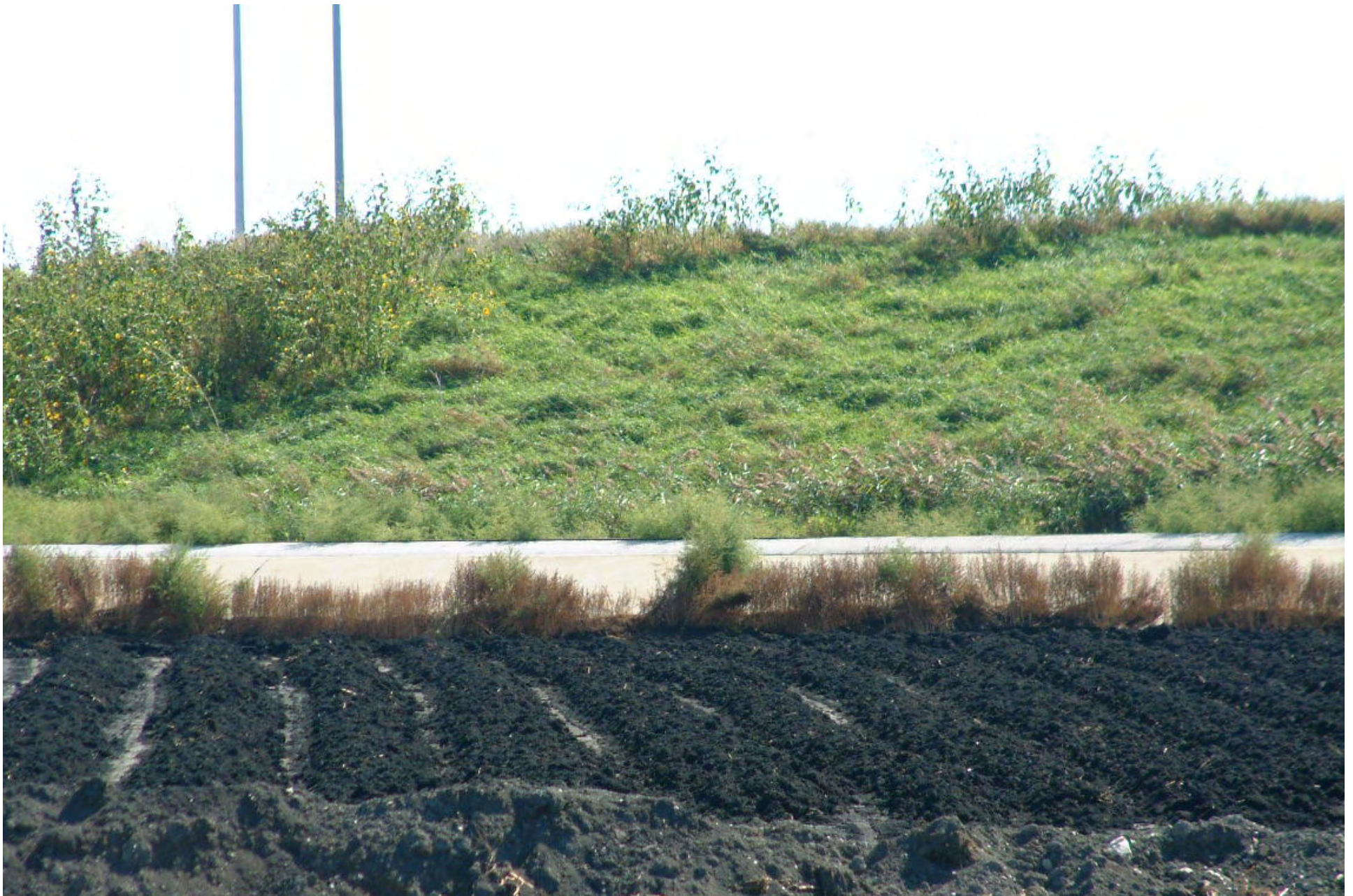
Windrowed Biosolids Resulting From Mechanical Agitation With Horizontal Auger (Brown Bear) During Air-Drying
