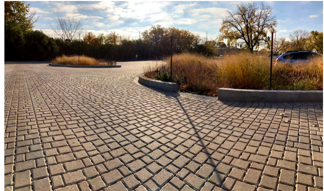
A permeable parking lot utilizing brick pavers and bioswale islands at Schuth’s Grove in the Forest Preserves of Cook County was completed in 2022 with funding from the MWRD through its Green Infrastructure Program.
