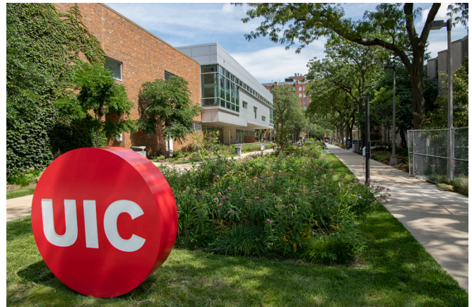
Arthington Mall Plaza at UIC stretches between Wolcott and Damen Avenues with 37,000 square feet of permeable pavement and rain gardens.
