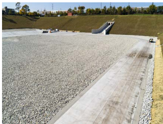
The Addison Creek Reservoir and the Addison Creek Channel Improvements are two associated flood control projects that will work together to provide significant benefits to communities along Addison Creek, including Bellwood, Northlake, Stone Park, Melrose Park, Westchester, and Broadview. The 600-acre-foot Addison Creek Reservoir will hold close to 200 million gallons of storage capacity and connect with the Addison Creek Channel.
