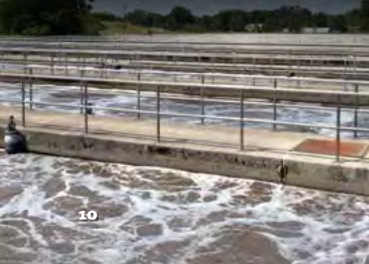
ACTIVATED SLUDGE TANK
