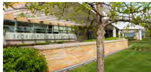
Skokie Police Station Headquarters can now retain 33,000 gallons of stormwater thanks to support from the MWRD.
