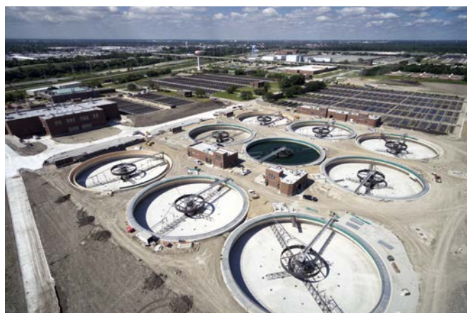
Capital Improvement Program projects, such as the primary settling tanks replacement at the Stickney WRP, aim to proactively modernize aging infrastructure.
