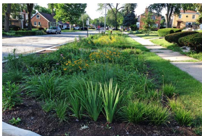
Left picture: Stormwater can be conveyed to rain gardens, such as the one in Blue Island, from downspouts. They are typically designed to drain ponding water within 24 hours. Right picture: Local businesses and volunteers with the Central States Water Environment Association sprang to action to partner with students at Skinner North Elementary School in Chicago to construct a rain garden.
