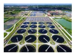
**ABOUT THE COVER** Final settling tanks at the Calumet Water Reclamation Plant (WRP) on the south side of Chicago. The facility can treat over 400 million gallons of wastewater per day.
