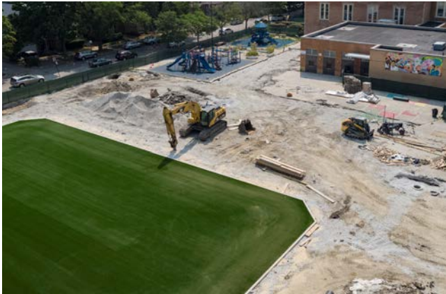
Construction on the Space to Grow schoolyard at Daniel Boone Elementary School.
