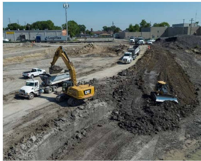
Excavation at the Addison Creek Reservoir in Bellwood, Illinois.
