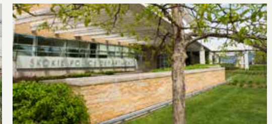
Skokie Police Station Headquarters can now retain 33,000 gallons of stormwater thanks to support from the MWRD.
