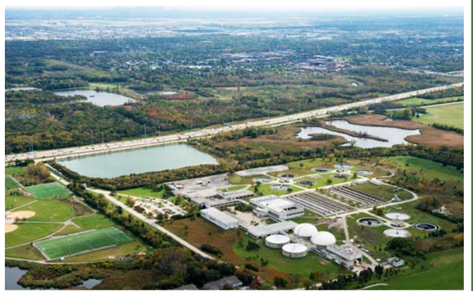
John E. Egan Water Reclamation Plant serves more than 160,000 residents in a 44 square mile area. In operation since 1975, the Egan WRP cleans an average of 30 million gallons of wastewater per day.
