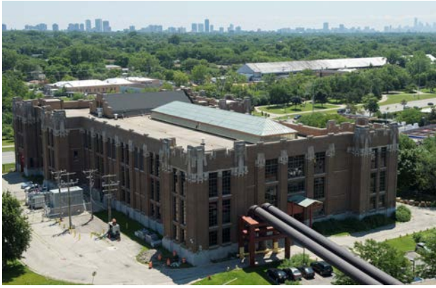
In 2020, the District will begin a $10 million rehabilitation of the steel spandrel beams in the pump and blower house at the O'Brien WRP.
