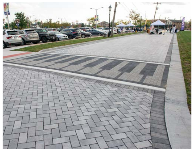
Permeable pavers on North Street, between Oak Park Avenue and 173rd Street in Tinley Park will provide 69,000 gallons of stormwater storage on site.
