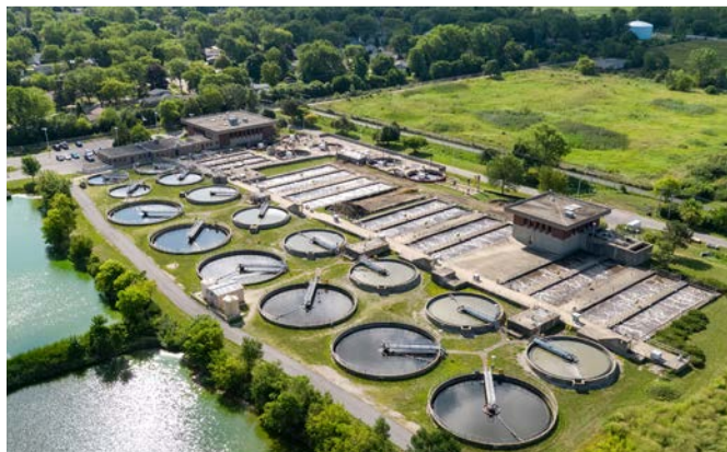
Hanover Park Water Reclamation Plant has been serving residents in northwestern Cook and DuPage County communities since 1963. The Hanover Park WRP serves more than 56,000 people within an 11.2 square mile area and cleans an average of 12 million gallons per day.
