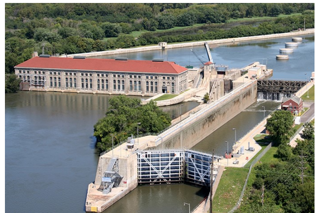
Lockport Powerhouse and Controlling Works. The Lockport Powerhouse generates approximately 40 million kilowatt hours of electrical energy annually, generating $1.2 million in revenue for the District.
