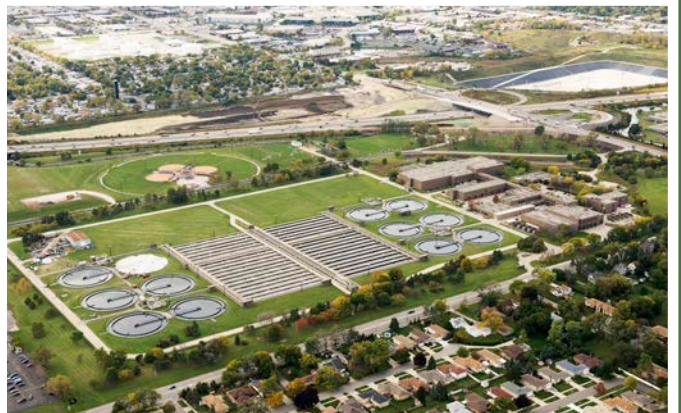
James C. Kirie Water Reclamation Plant opened in 1980, making it the newest of the MWRD's seven wastewater treatment plants. The 108-acre Kirie plant serves a population of about 264,000 residents in a 65.2 square mile area to clean more than 50 million gallons of wastewater per day.
