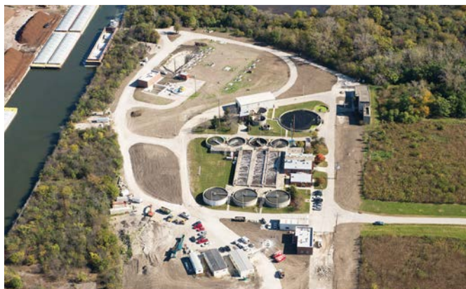
Lemont Water Reclamation Plant is a small but industrious MWRD facility that provides wastewater treatment for a service area of more than 20 square miles that includes nearly 23,000 people in the village of Lemont. It opened in 1961 and cleans an average of 2.5 million gallons of wastewater per day.
