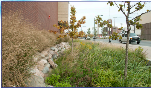
Bioswale – green infrastructure solution to capture stormwater runoff
