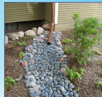
Disconnected downspout
