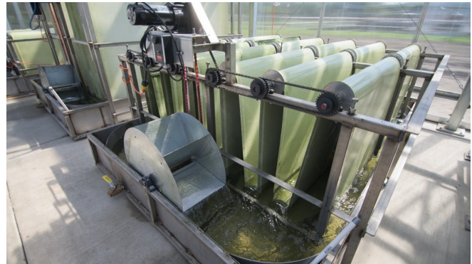
Algae naturally uptakes phosphorus and nitrogen from water to support its growth through photosynthesis, utilizing the sun as its energy source here at the MWRD’s greenhouse at O’Brien Water Reclamation Plant.
