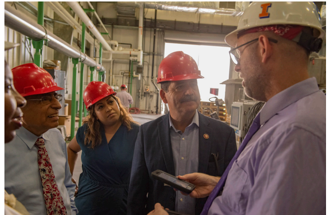
MWRD Commissioner Frank Avila, State Rep. Celina Villanueva and U.S. Jesús G. “Chuy” García look on as MWRD Managing Engineer Joe Cummings and Senior Engineer Debra Hill lead them on a tour of the Stickney Water Reclamation Plant’s nutrient recovery facility, where the MWRD recovers phosphorus and nitrogen from wastewater streams and converts it into a slow-release fertilizer.
