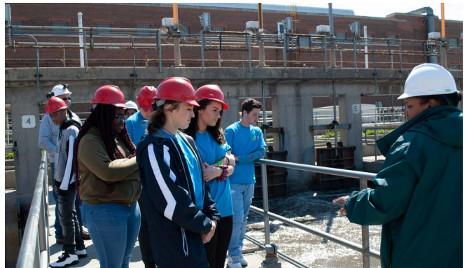
Take our Daughters and Sons to Work participants see treatment tanks up close at the MWRD's Stickney Water Reclamation Plant.
