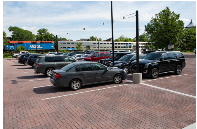
A new permeable parking lot in Riverside, partially funded by the MWRD, will give Metra commuters a place to park and ride and also a place to absorb more stormwater that will protect the community from flooding.
