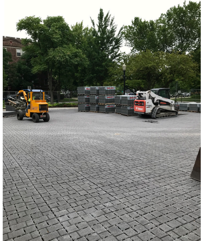
The permeable parking lot under construction earlier this year.
