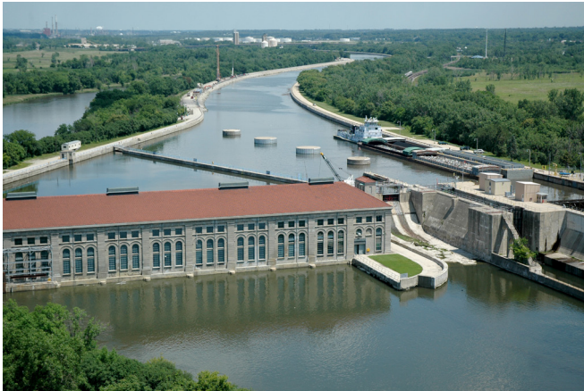
Lockport Controlling Works and Powerhouse
