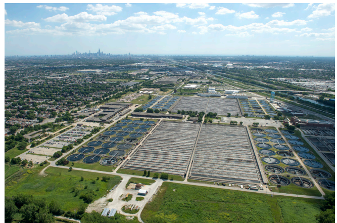
The MWRD's Stickney Water Reclamation Plant transforms as much as 1.2 billion gallons of water per day, serving 2.3 million people from central Chicago and 46 suburban communities.
