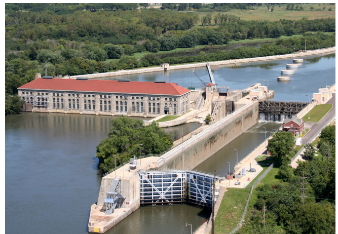
The MWRD's Lockport Powerhouse and Controlling Works are undergoing a major rehabilitation project that will rely on the manpower and skill of the Will and Grundy Counties Building Trades Council and Three Rivers Construction Alliance.
