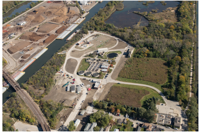
The MWRD's Lemont Water Reclamation Plant is home to a new energy efficient turbo blower that keeps air flowing to treat water and will save the MWRD nearly $27,613 in energy costs annually.
