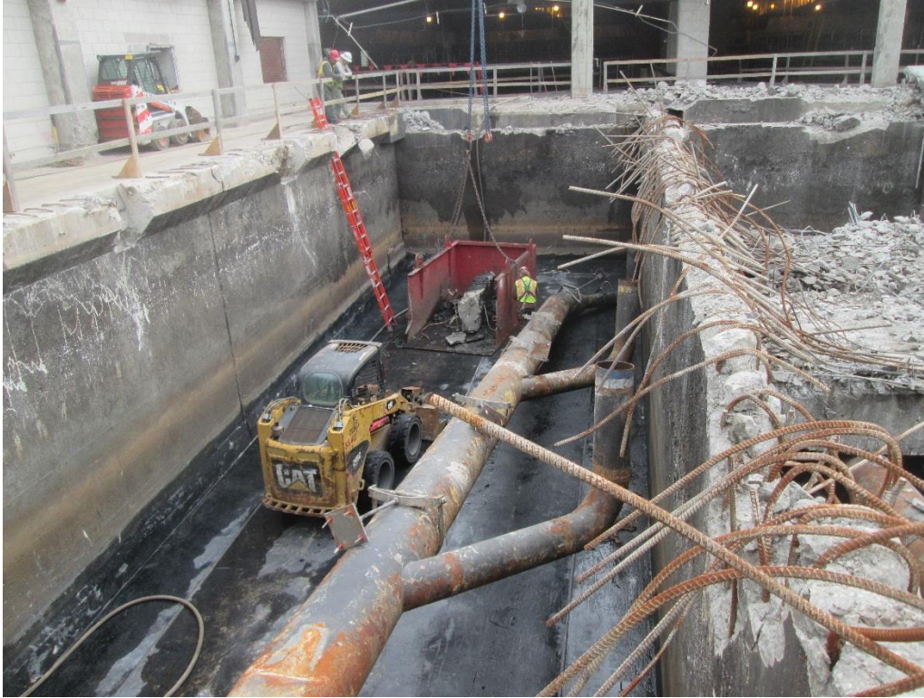
a) Looking south
