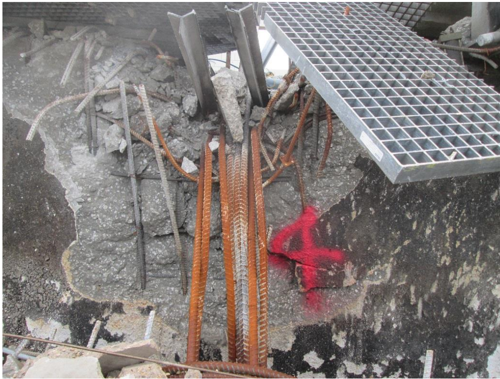
a) Top continuous reinforcing bars
