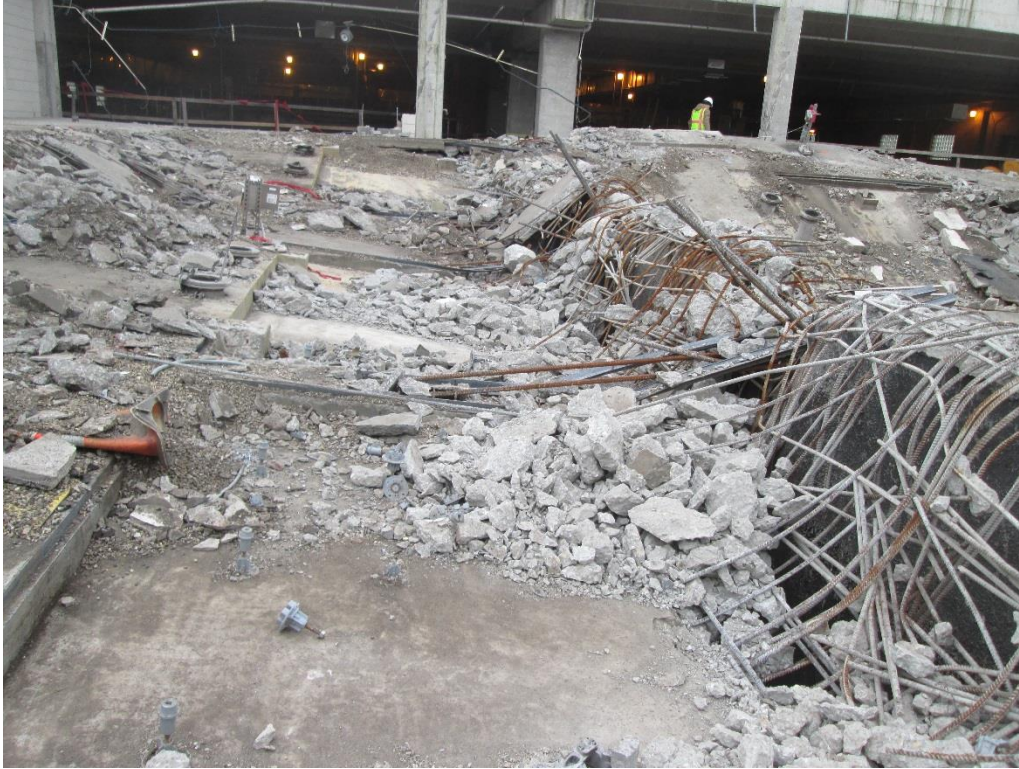
a) Overall view
