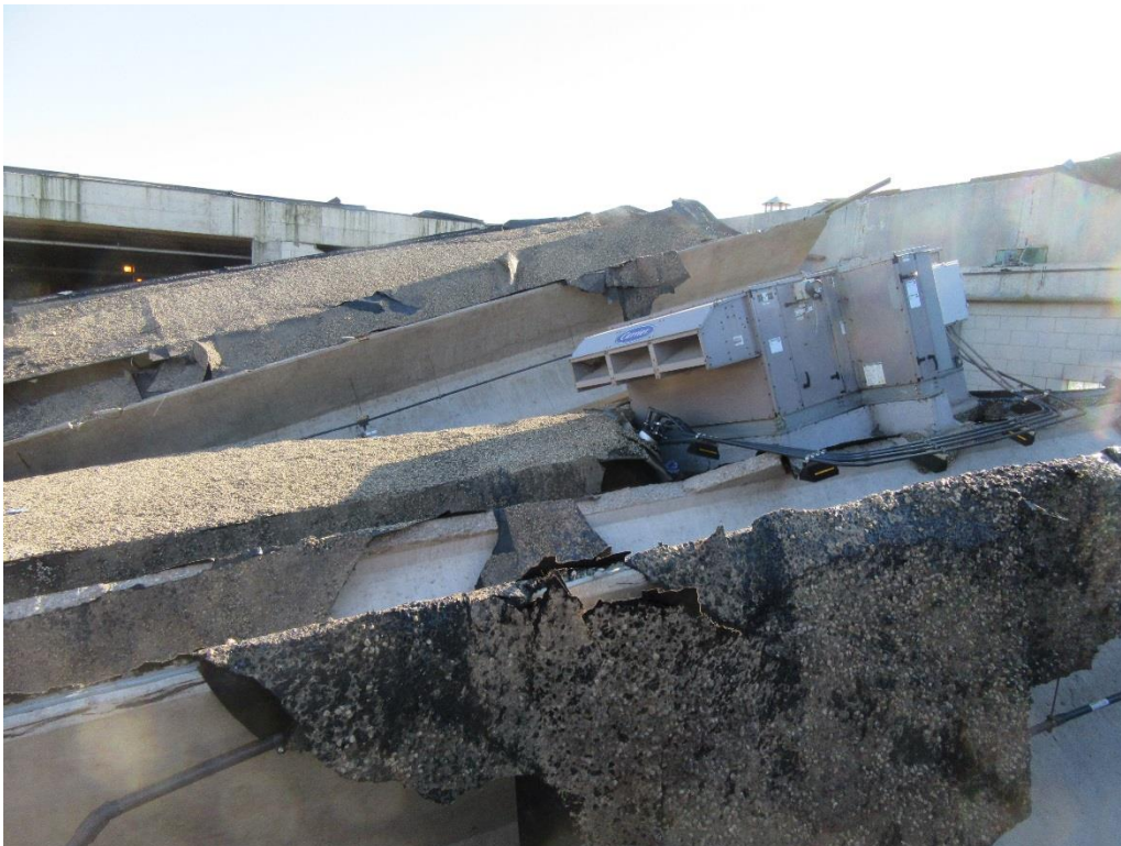
b) Looking southwest
