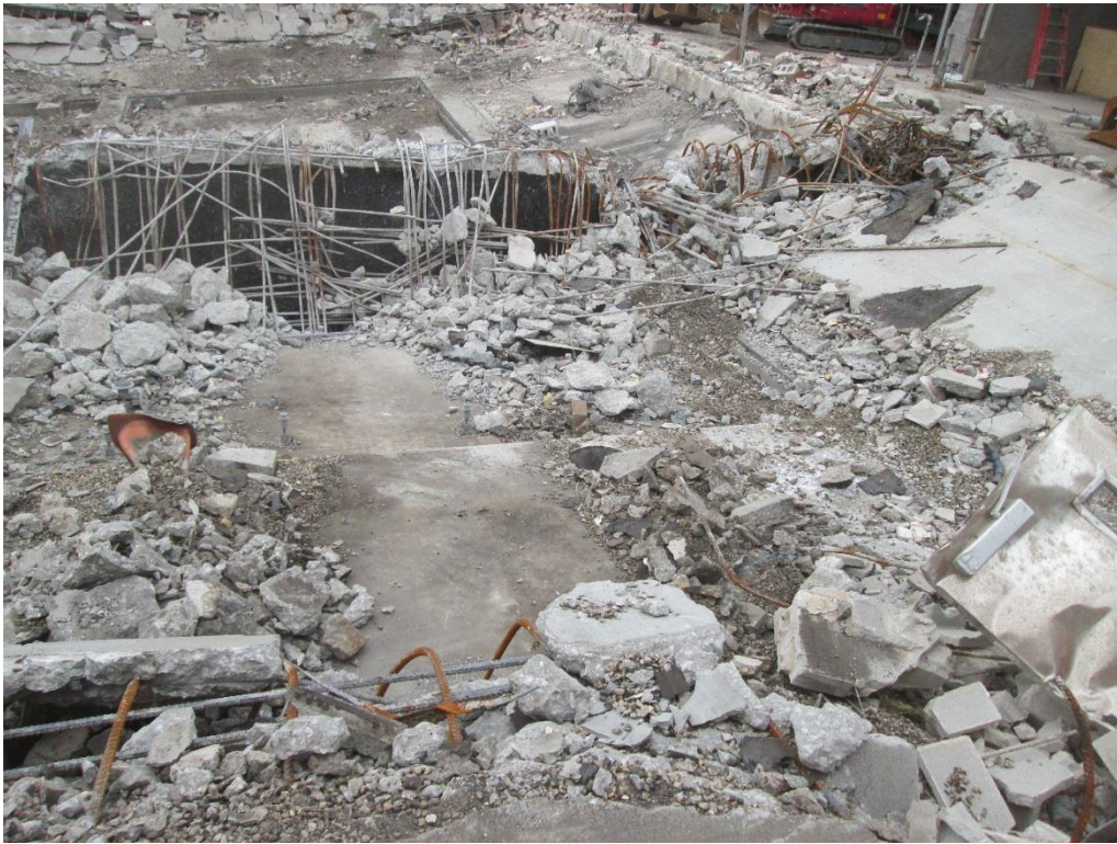
Figure 24. Intact floor slab over center portion of east tank looking west
