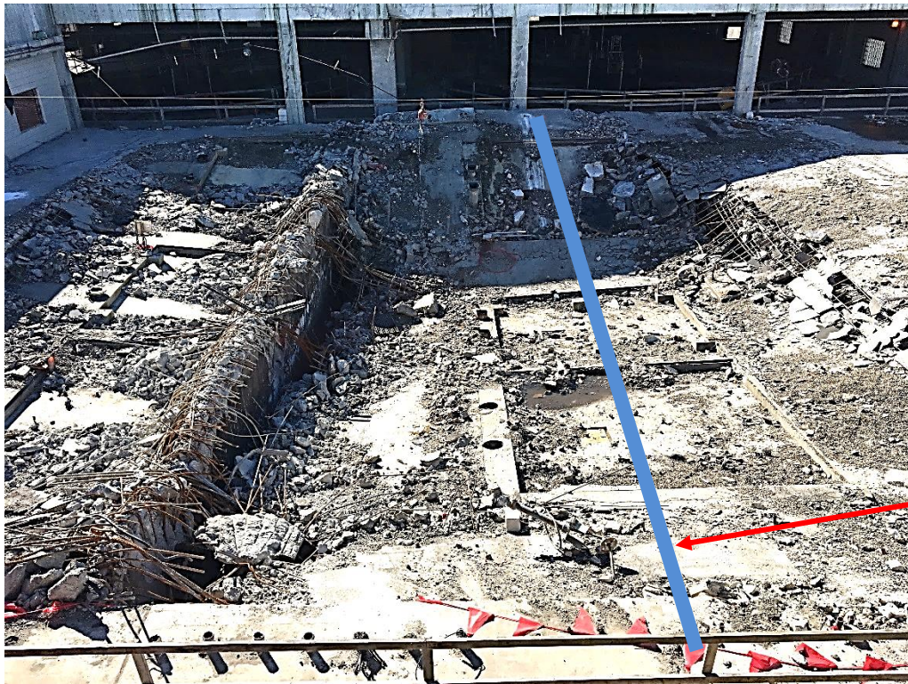
Figure 26. GBT Room floor slab over center and west tanks
