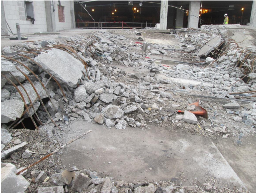
a) Overall view
