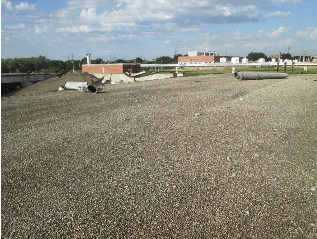
a) Overall view
