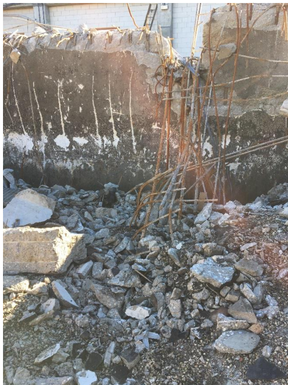
Figure 23. Damaged GBT Room floor slab and beams over the center tank on the west side of interior wall between the east and center tanks
