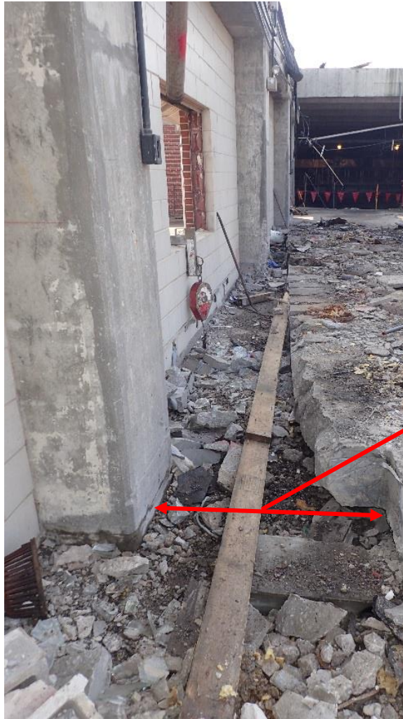
Figure 19. Floor slab movement at east wall, looking south
