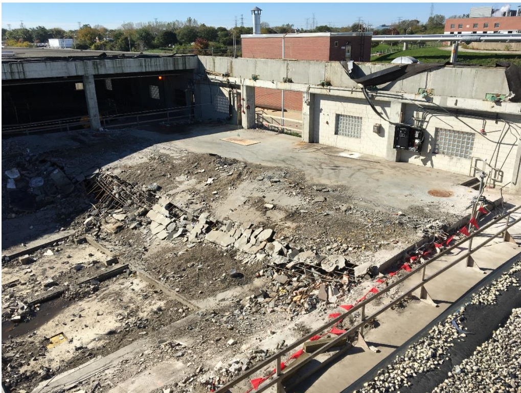
Figure 25. West side of GBT Room floor slab
