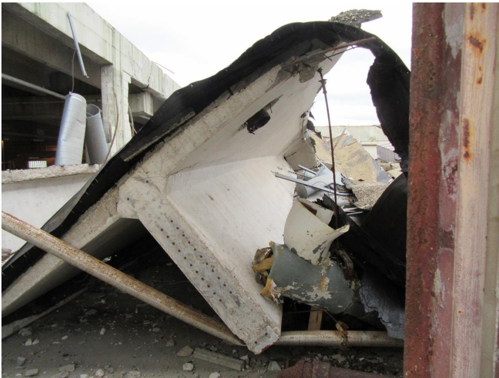
Figure 6. End view of precast prestressed single tee roof beam
