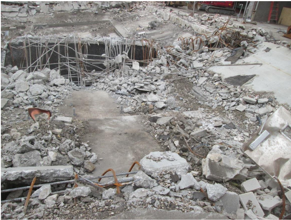
b) Close-up view looking west
