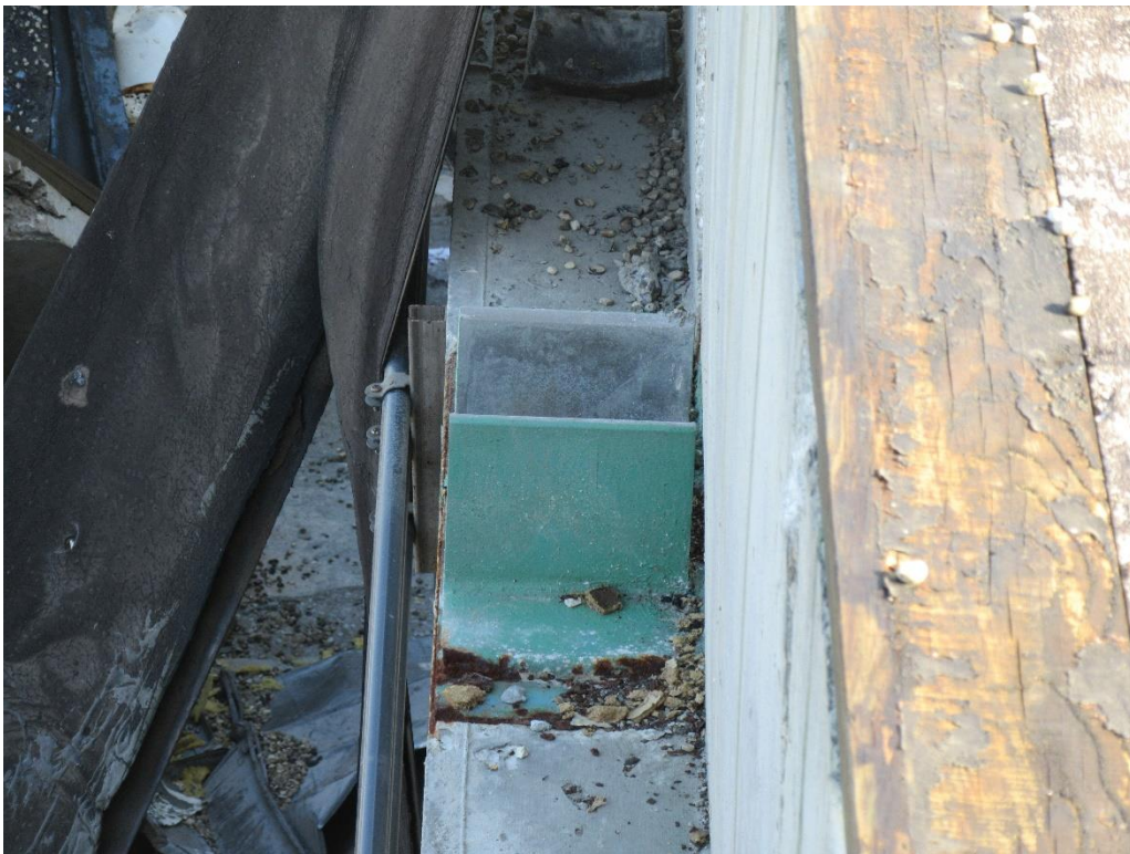
Figure 8. Single tee roof beam bearing location at east wall of GBT Room
