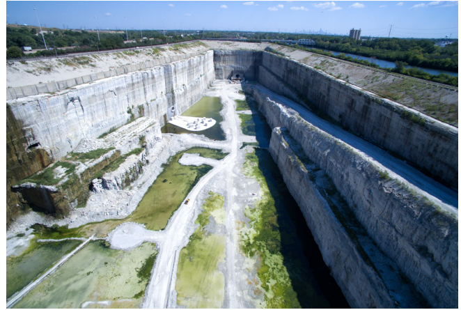
Stage I of the McCook Reservoir benefits 3.1 million area residents and now many more will hear about its impact after the Water Environment Federation bestowed it with a Project Excellence Award.
