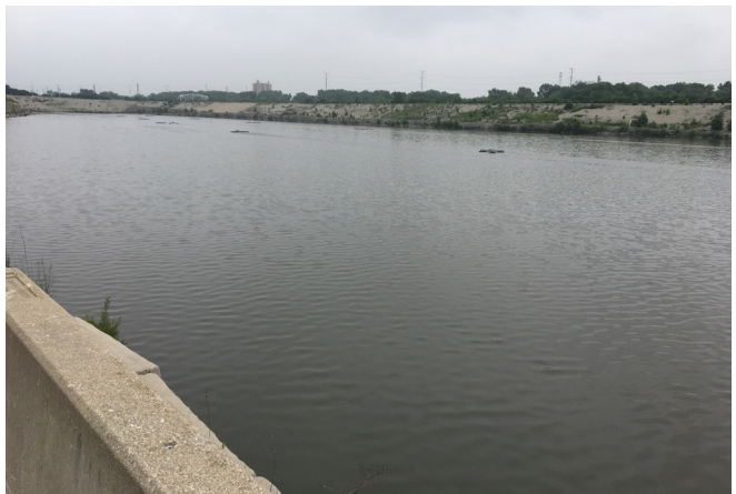
The McCook Reservoir Stage I filled in June, demonstrating a fully operational system retaining water that formerly discharged to the Chicago Area Waterway System or ended up in basements of homeowners and businesses. Another 6.5 billion gallons of capacity will become available through Stage II.
