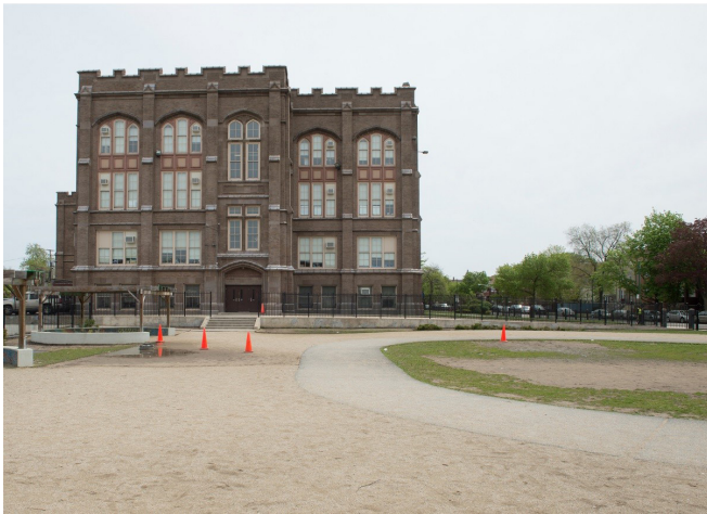
Davis School, before.
