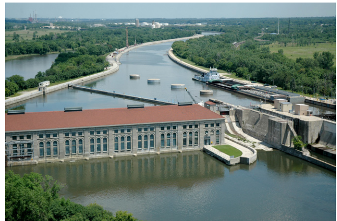
Lockport Powerhouse, Lockport, Illinois.
