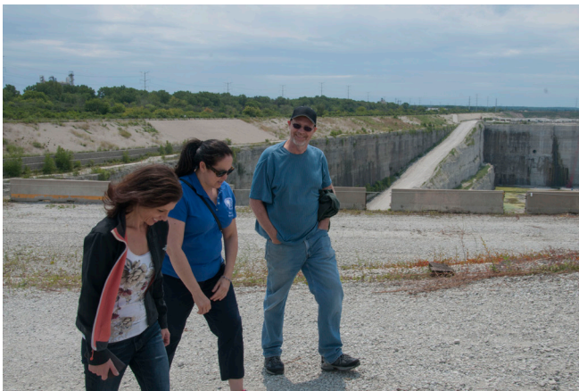
MWRD President Mariyana Spyropoulos (center) discusses the McCook Reservoir, part of the MWRD's Tunnel and Reservoir Plan, during a public tour.
