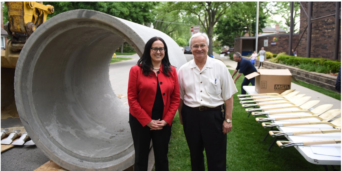
Metropolitan Water Reclamation District of Greater Chicago President Mariyana Spyropoulos and village of Niles Mayor Andrew Przybylo stand before some of the giant storm sewer infrastructure that will be installed to provide flood relief to Niles.
